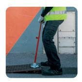
STEP 2 Magnetize the edge, lift it slightly and pull it by sliding the plate on the ground
